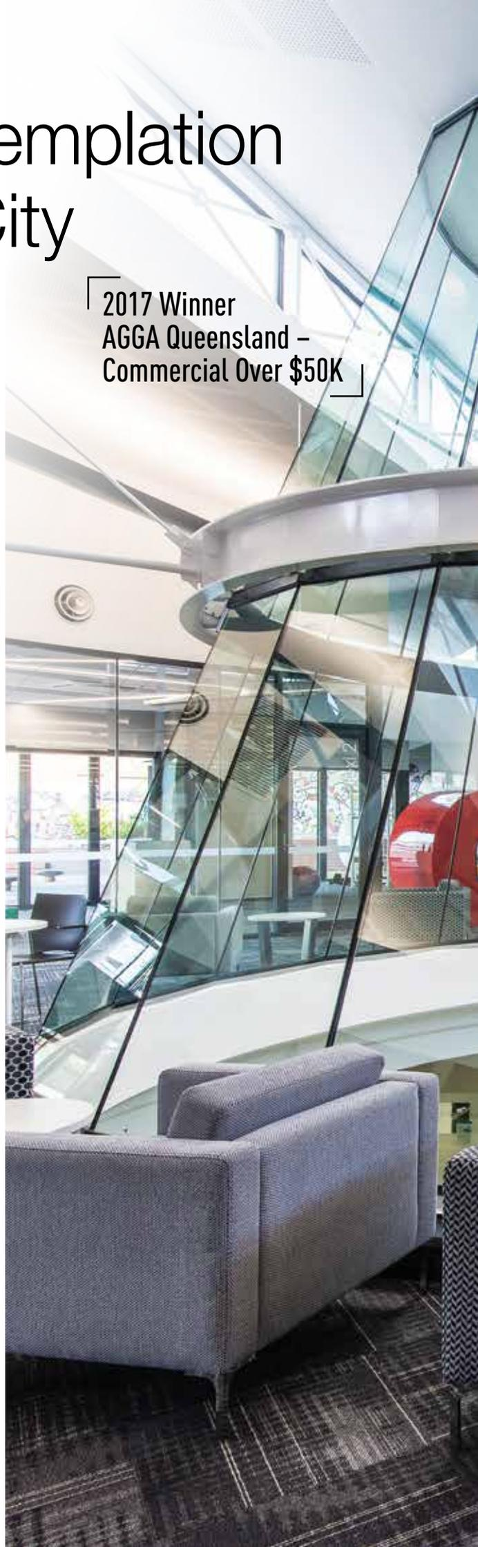
“ Before any of the glass was installed, the builder had to pre-load the centre ring that formed the base of the dome, which was strapped to the lower ground shopping arcade floor ”
